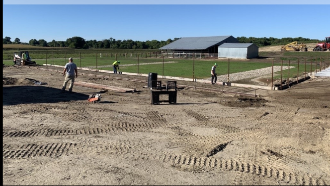
Ag. Waste Pit 1 - Before
