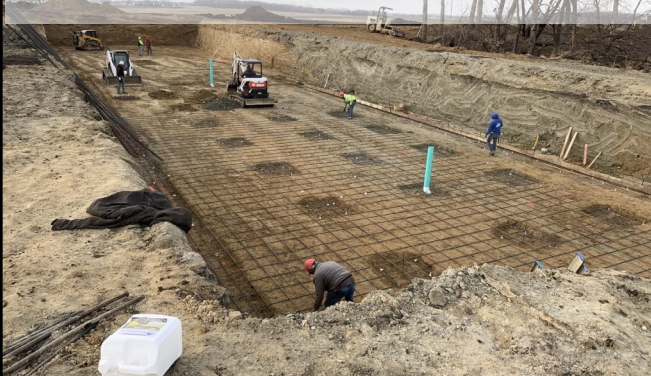
Ag. Waste Pit 2 - Before
