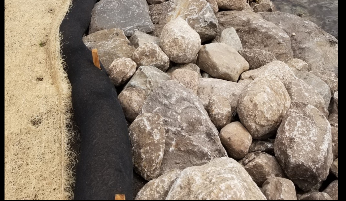
Shoreline Project - After
