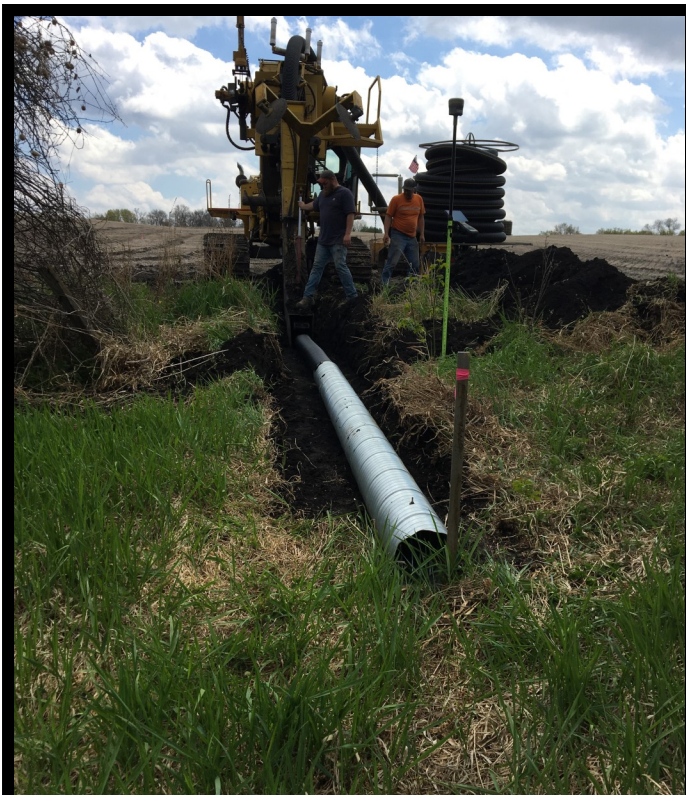
Tile Outlet Installation
