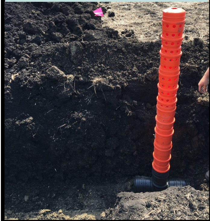
Intake assembly Installation
