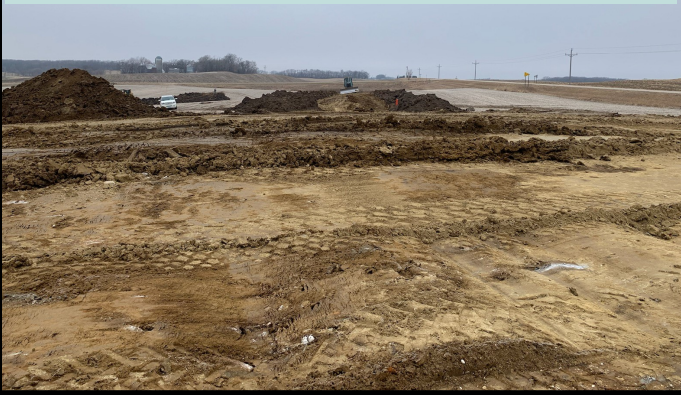
Completed WASCOB with intake
